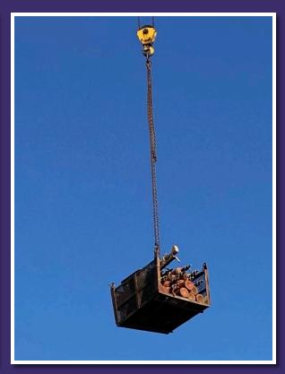
Among other jobs for which the shipyard's riggers and crane were essential was removing CO2 cylinders from the hold
